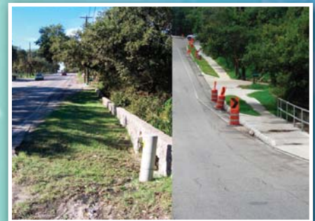
Without Public Works | With Public Works
